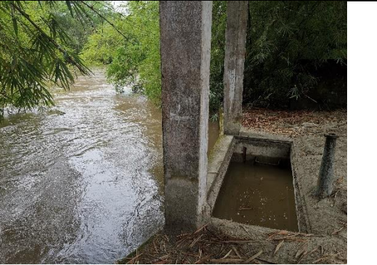
San Alberto River Catchment System
