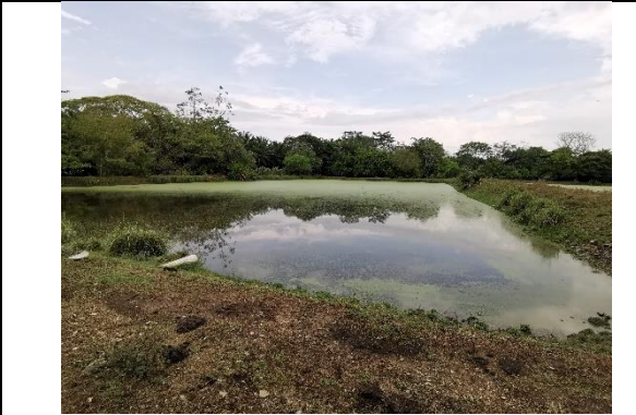
Industrial Wastewater Treatment System - Lagoon Systems
